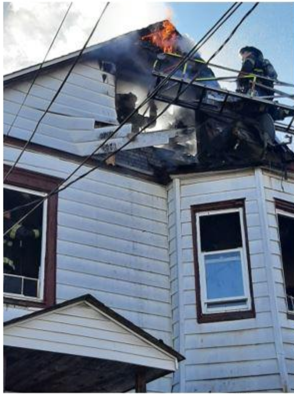
February 26, 2021 – Fire at 384 South 19 th Street, Newark
